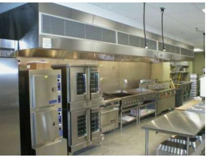
At the near end of the cook line is a stacked steamer. From this angle we can see that the deeper 54" hood will capture steam when the doors of the steamer open.
