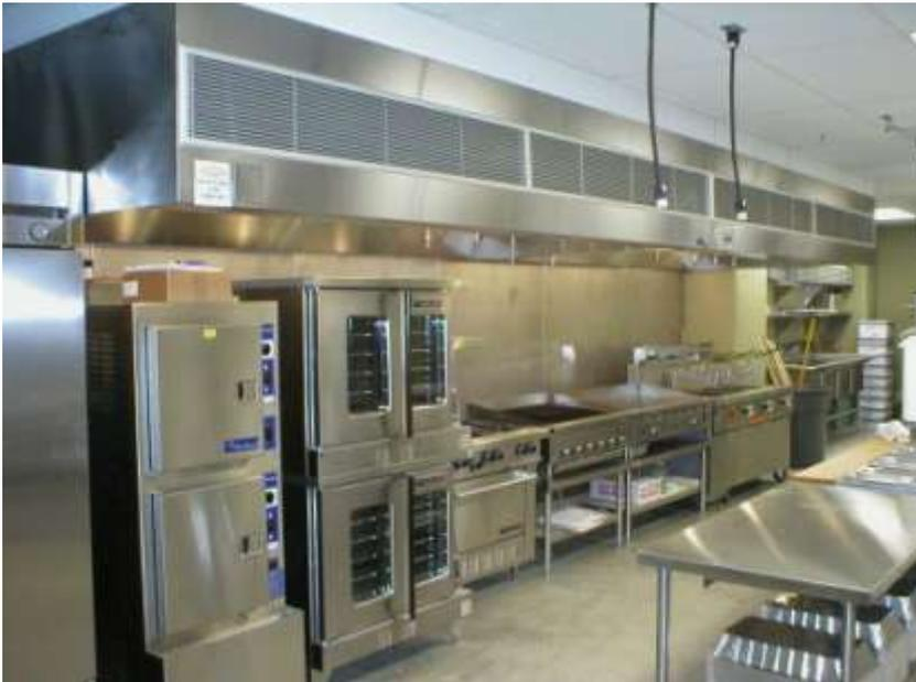
At the near end of the cook line is a stacked steamer. From this angle we can see that the deeper 54" hood will capture steam when the doors of the steamer open.
